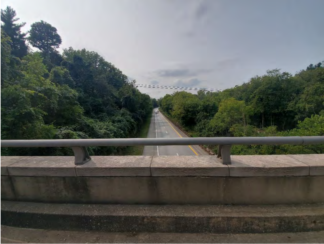
Photo No. 3 – View of I-64 WB lanes looking east from Alta Vista Road overpass
