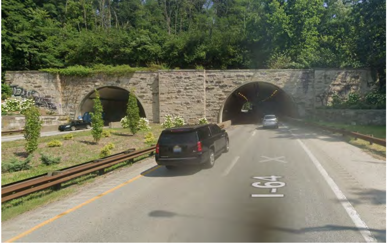
Photo No. 7 – View of west portal of Cochran Hill Tunnel
