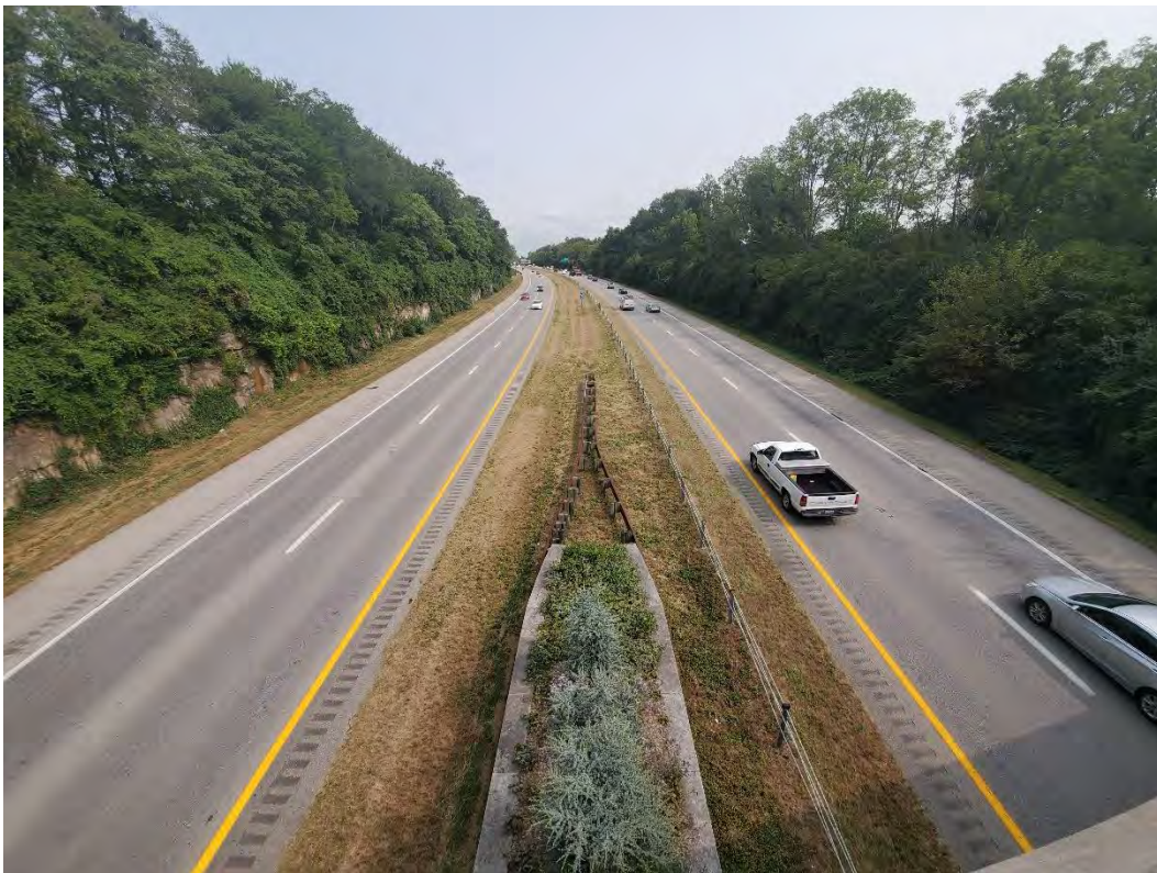
Photo No. 2 – View of I-64 looking east from Pee Wee Reese Road overpass
