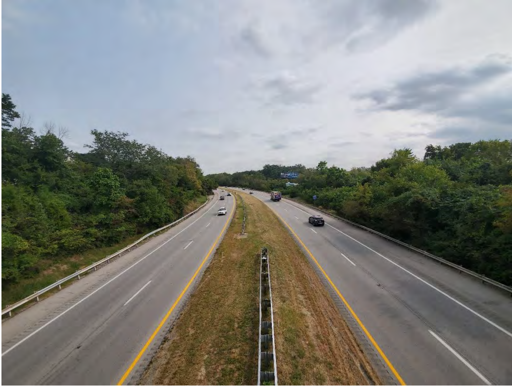
Photo No. 1 – View of I-64 looking east from Payne Street overpass
